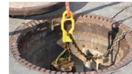
Lift a pump with chain gripper
